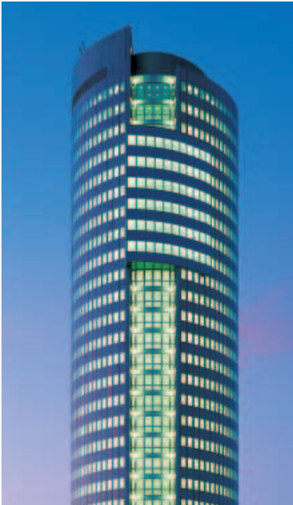
Florido tower, Vienna, Austria Florido Tower, Vienna, Austria
