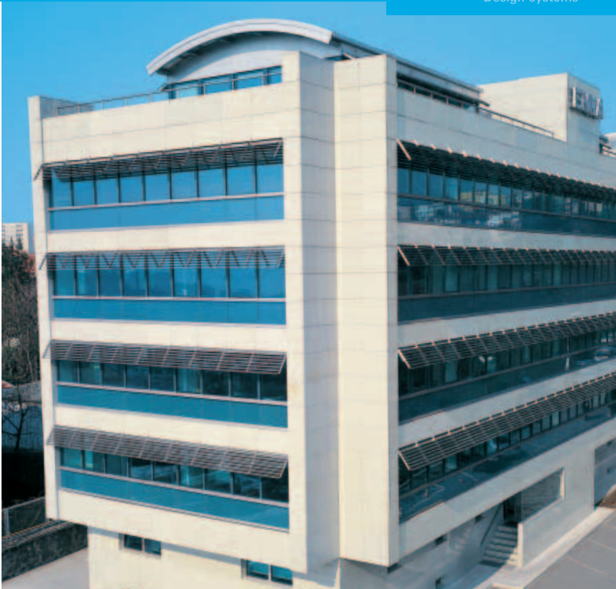
Enka Building, Istanbul, Turchia Enka building, Istanbul, Turkey
