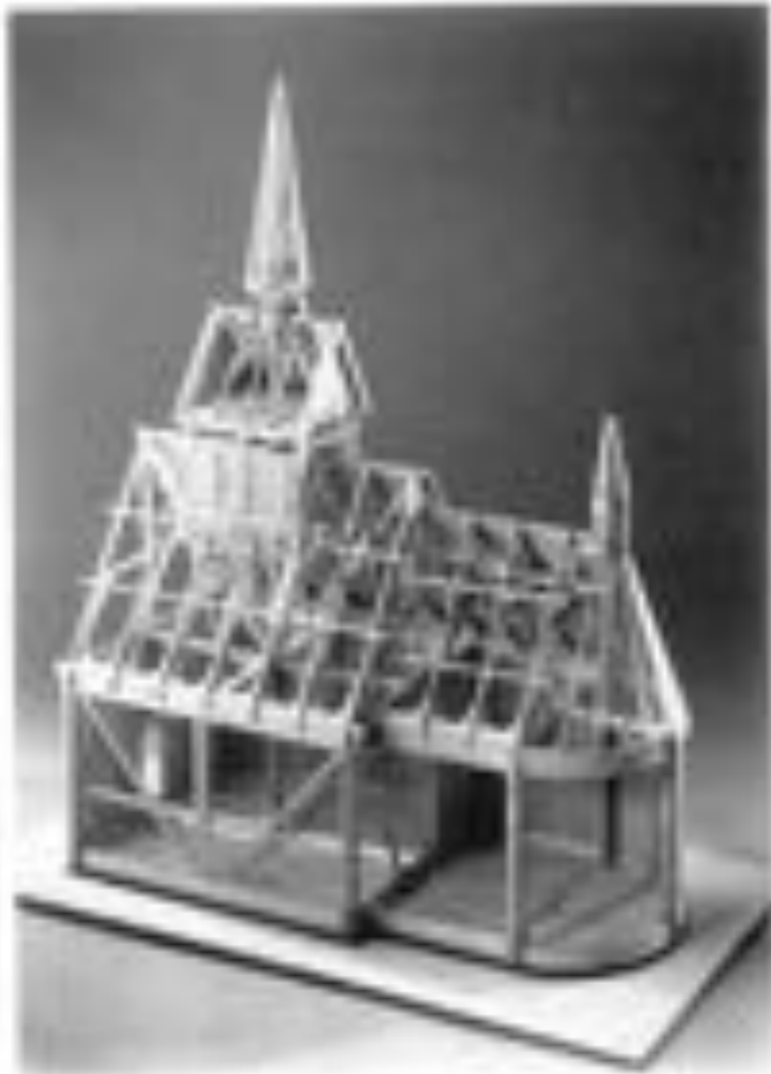
Model of a Gothic building showing the truss system of the roof and the spire.
